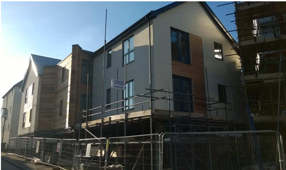
Affordable flats under construction 2017, Long Street, Dursley.
