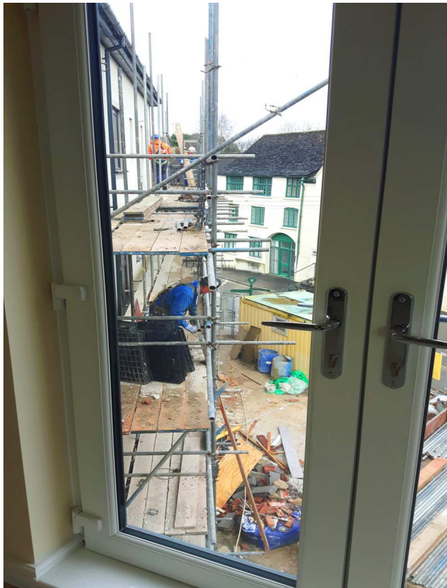
Affordable flats under construction at Dursley, 2017
